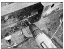
After the pilot marks were made, we withdrew the CPP bracket away from the frame before drilling. This was to avoid accidentally "hogging-out" the CPP bracket.
