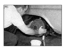
After properly setting the car on jackstands and removing the rear wheels, we proceeded to remove the drum and all of
