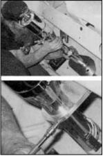
Now the column was set into place, and the column drop was tightened up.
