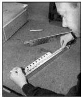
2..The side-to-side mounting brackets are long and can be trimmed to fit. Next transfer the dimension to the bracket with a felt tip marker.
