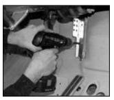
19..As was mentioned earlier, the mounting brackets can be bolted to the firewall. Simpfy drill holes and attach the mounting brackets with nuts, bolts and lock washers.
