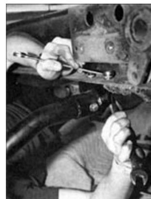
11. Likewise, the transmission crossmember is secured to the bottom channels of the framereils
